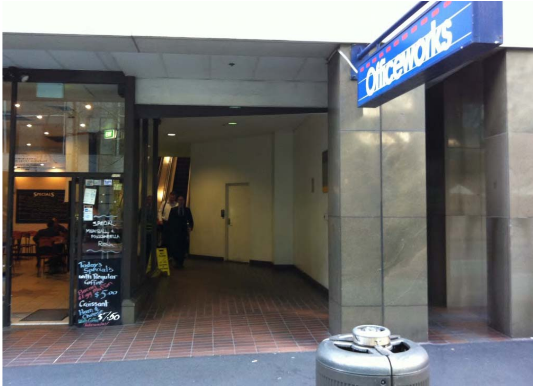
Figure 4 – existing mid-block connection (Clarence Street)
